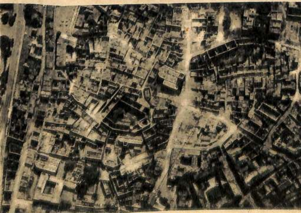
The center of what used to be Mainz, after the R.A.F. came over.
