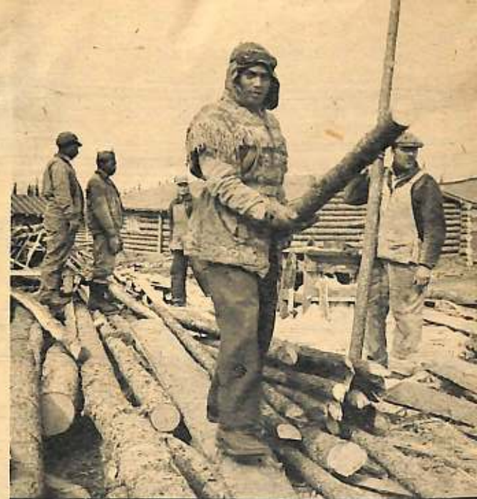
This Negro GI from an Engineer service unit helps cut rafters for log cabin barracks in a north Canadian construction camp. He's sporting an Indian parka.
