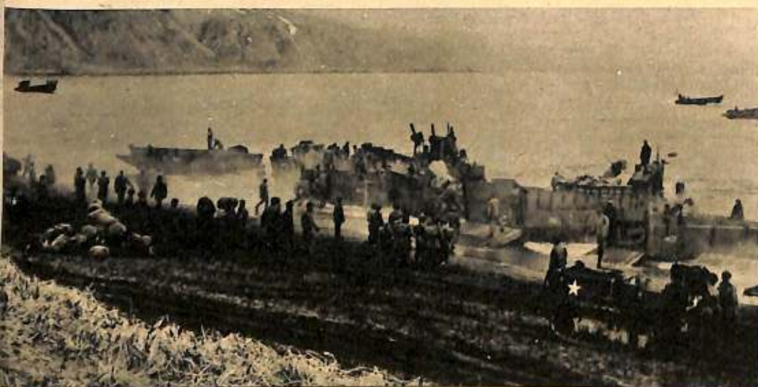
Off the landing barges to the singularly unpleasant soil of Attu in the Aleutians come the first wave of troops that eventually ousted the Japanese from the island. Evidently engineers, they brought their bulldozers with them.
