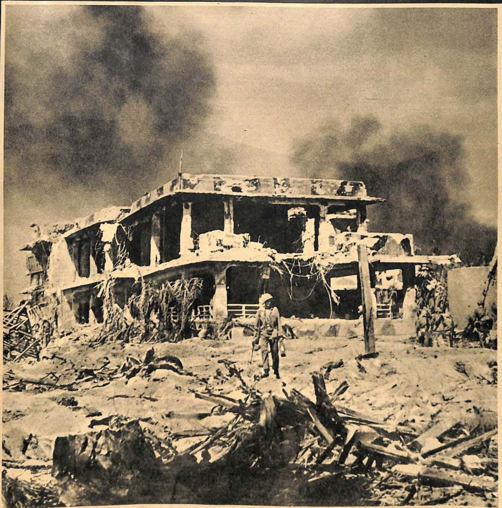
THE WALLS OF THIS POWER PLANT ON ENNUBIRR ISLAND WERE TWO FEET THICK BUT THAT WASN'T THICK ENOUGH TO TAKE THE NAVY'S SHELLING.
