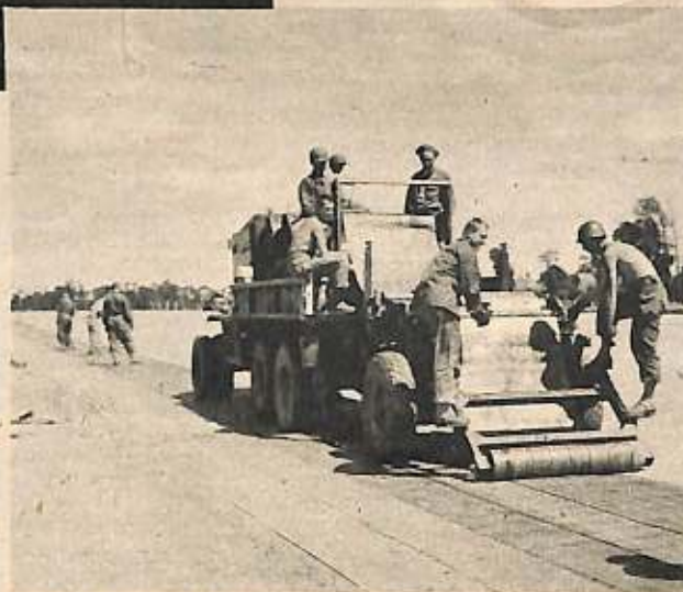
53 The Ninth Air Force needed air fields in France. Engineers were there to lay them out.
