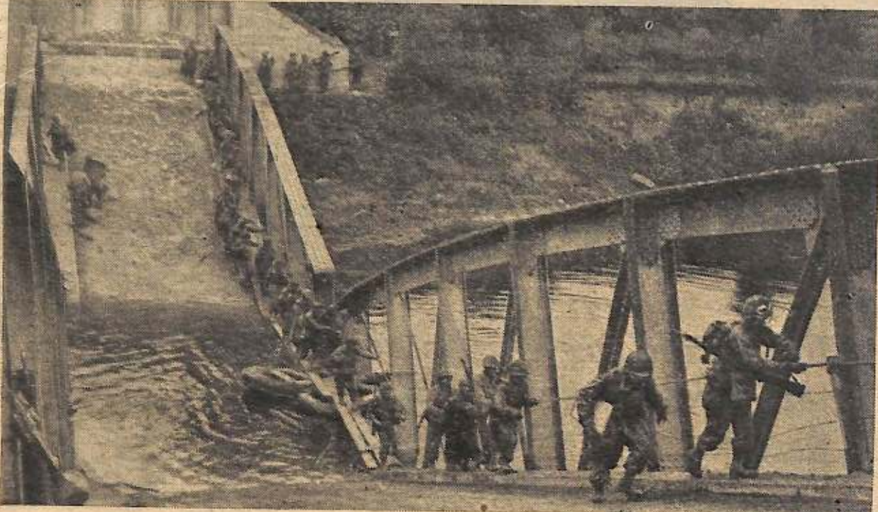
The Germans dynamited this bridge across the Marne River at Mareuil sur Ay, but U.S. infantrymen cross it anyway.
