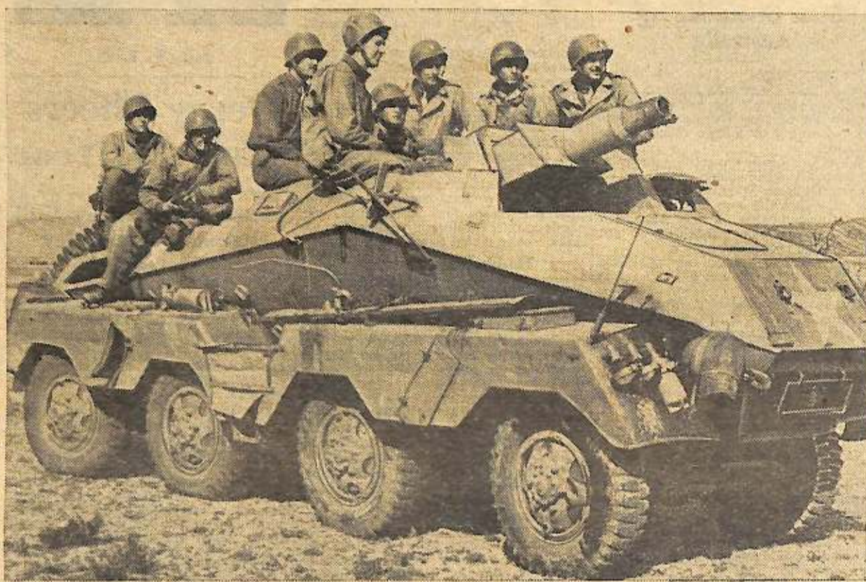
This German tank destroyer was captured by the U.S. Second Corps from the 10th German Panzer Division during a battle in Tunisia. As soon as a U.S. Army ordnance crew made minor repairs and painted a star on it, Yanks took it back into action against the Nazis. It has a 75-mm. cannon and dual controls, operating both forward and backward.
